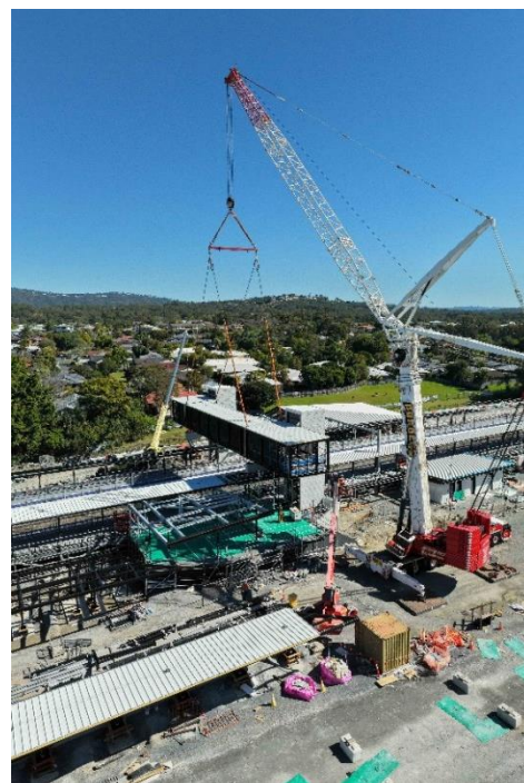
Above: Installation of the pedestrian overpass, connecting inbound and outbound station platforms
