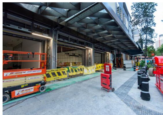
Image above: Lot 3 canopy works progressing
