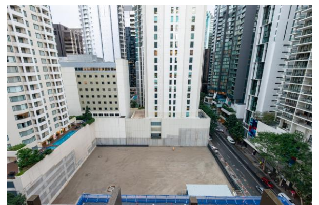
Image above: Remediated Lot 2 site
