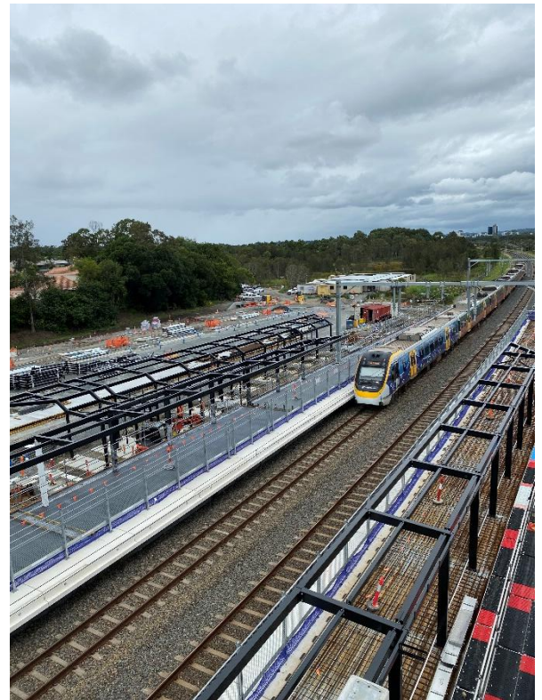
Above: station platform construction is underway.
