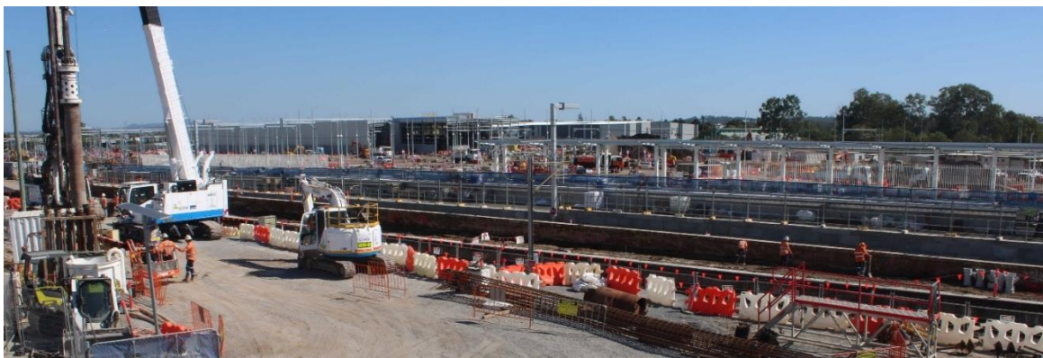
Above: Moorooka station entry piling works April 2026
