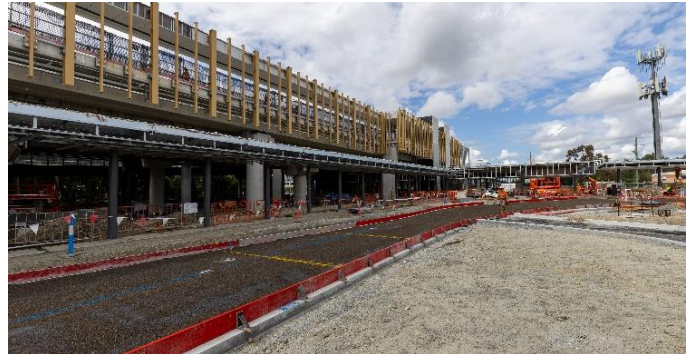
Pictured: Bus bay and platform construction
