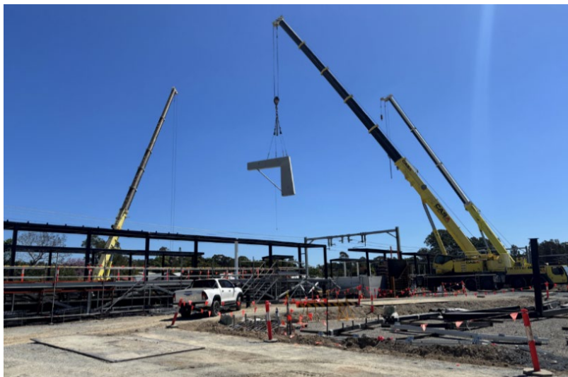
Above: station platform construction, including pre-cast column installations
