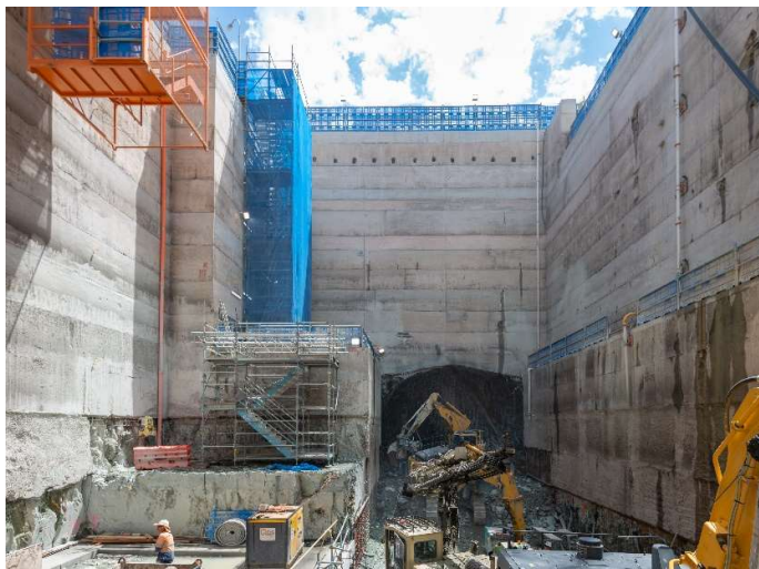
Image: The bottom of the services building shaft. Excavation of the tunnel connecting this shaft to the new underground cavern is underway.
